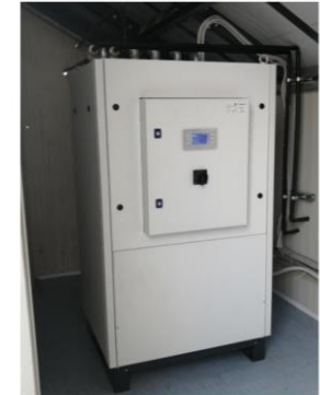
Technical innovation: patented zeolite coating technology, reducing the unit's volume and cost by about two times
